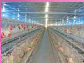
Poultry House Project
